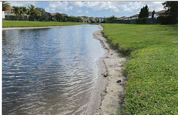
Photo 9: Lake 3 south side erosion with 1-2' drop off
