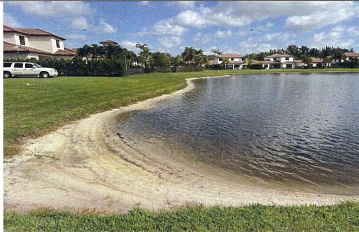
Photo 11: Lake 3 NW side erosion with 1-2' drop off
