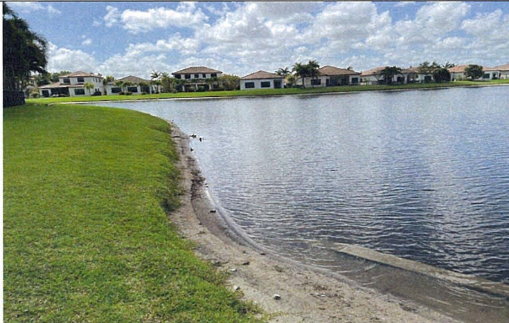
Photo 10: Lake 3 NW side erosion with 1-2' drop off
